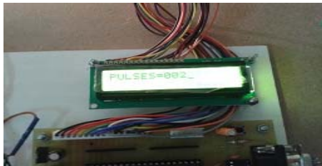
Fig.10: LCD showing energy consumption data
